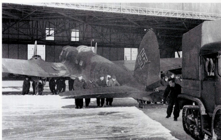
ABOVE: An He 111 of KG 55 is towed from its hangar by a half-track vehicle during the winter of 1940/41. By this time the paint finish has become extremely weathered which has resulted in the camouflage pattern of the two greens (RLM 70 and 71) appearing more visible than usual.
